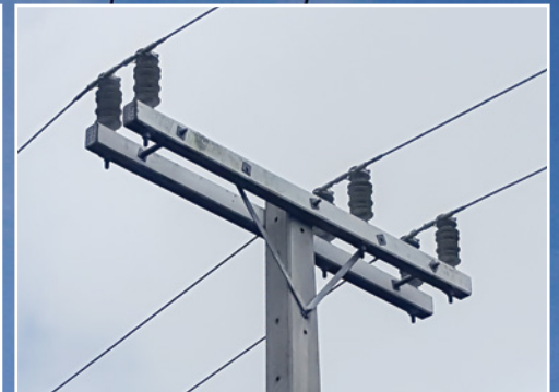
11kV Polymer Posts - King Country
