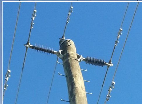
66kV Polymer Posts - Southland
